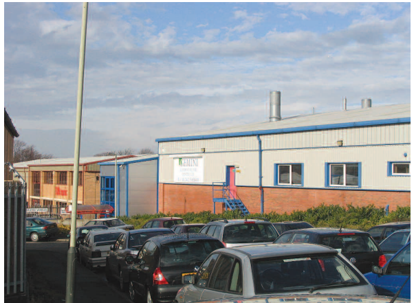
Full management of extensive industrial building in Cheltenham.
